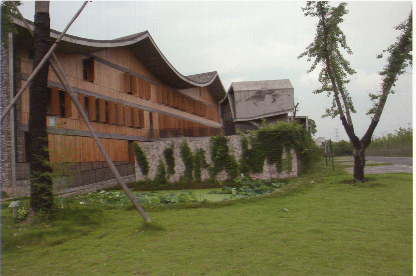
Vista completa de la fachada de madera con los corredores parcialmente abiertos al exterior del edificio 19, aulario de la Escuela de Moda. Full view of the wooden façade with the corridors partially open to the exterior of building number 19, Fashion Design school classrooms.
